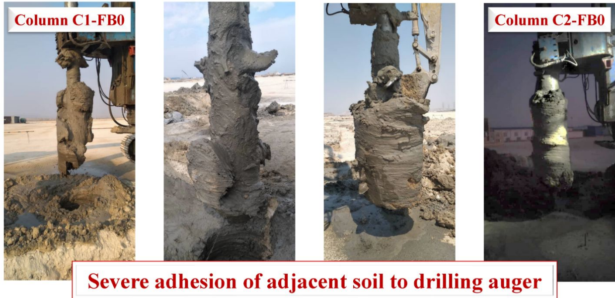
Fig. 9. Visual condition of auger FB-0 (without free blades) after drilling DSM columns
