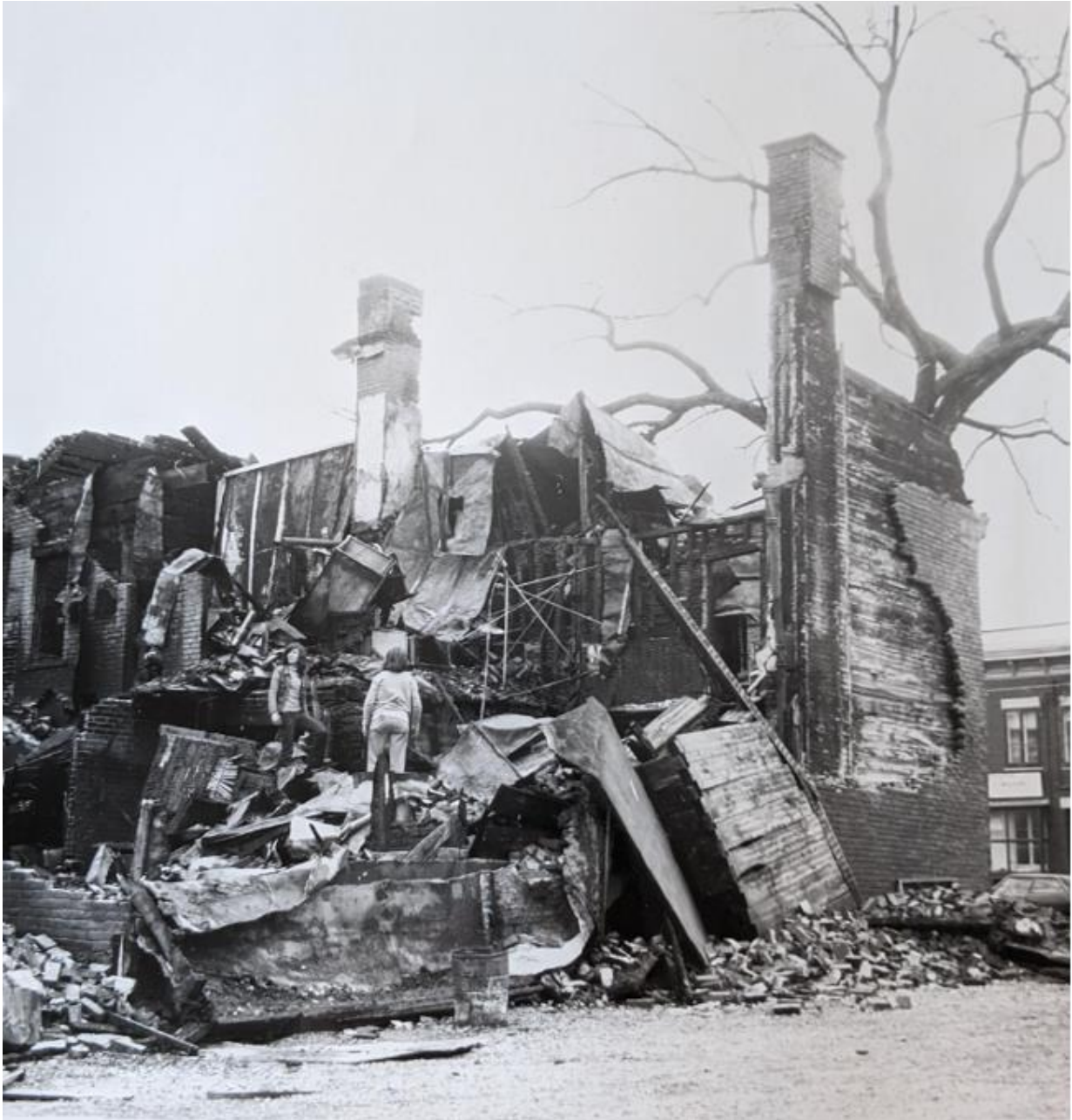
Figure 23: Two Saint-Jacques ward residents survey the damage caused during the Red Weekend. Plessis Street, 4 November 1974. VM007-Y-1-D37, AVM.
